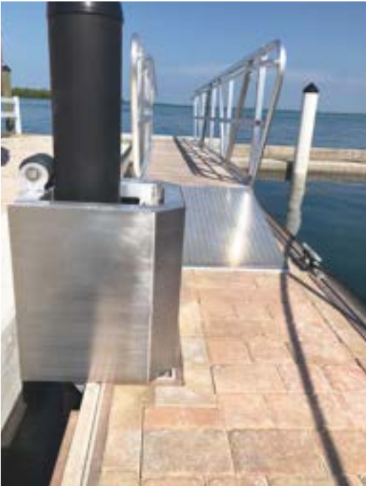
Protective Cowling Constructed with 6061-T6 Aluminum
