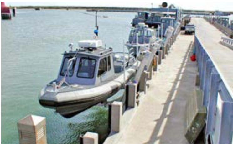
Client: Texas Navy Base Products: (3) Elevator Lifts
